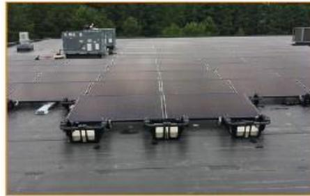
All wiring managed under module, FR510 chassis or in listed raceway.
